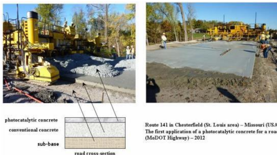
Fig-2: Cross-sectional view of two-lift paving, showing the base layer and photocatalytic top layer
