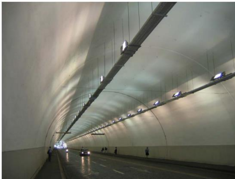
Fig-3: Photocatalytic coating applied to a tunnel's internal surface, maintaining cleanliness and air quality
