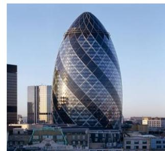
Figure 1 - Example of Diagrid Structural System
