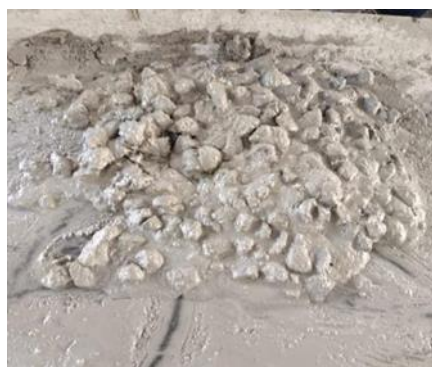
Fig 5.2: Mixing of Concrete
