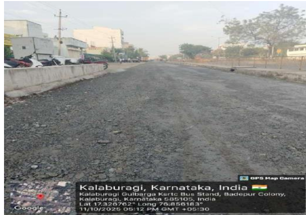
Fig:1.3 due to construction of service road
