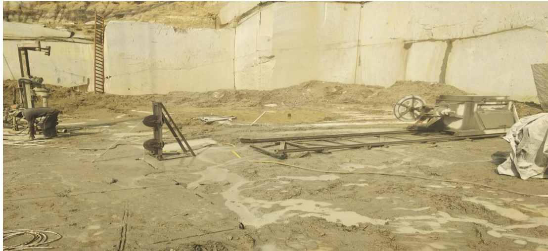
Figure 7-Diamond wire saw cutting blind cut
