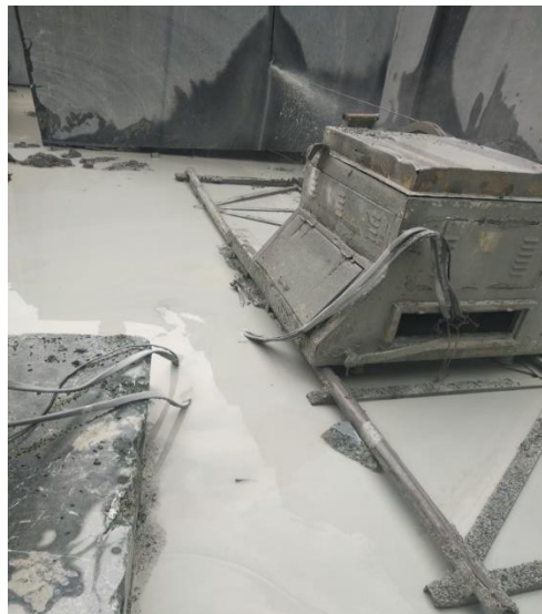
Figure 4 -Fixed speed diamond wire saw machine cutting vertical cut
