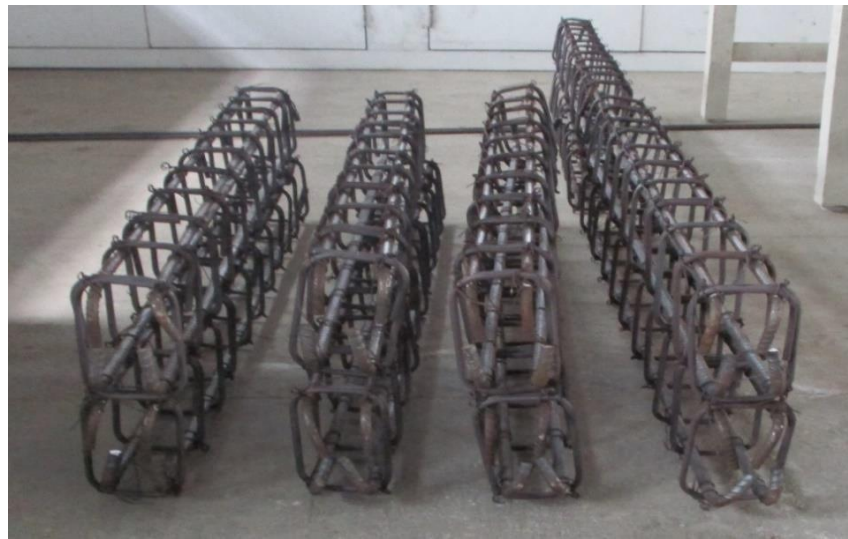
Figure 12 : Tied reinforcement cage of beam
