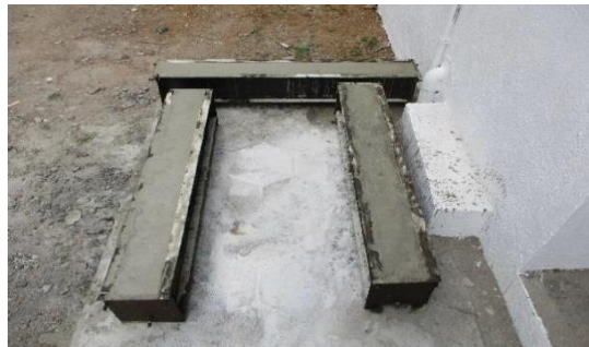
Figure 13: Various stages involved in casting of beams
